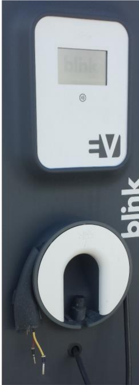
Inoperable Level 2 EVSE at San Diego State University
