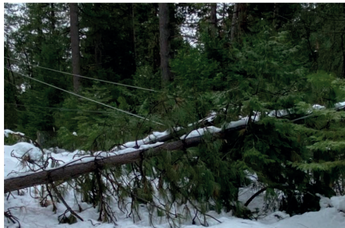
Figure 4: PG&E Covered Conductor Effectiveness – Example 3
