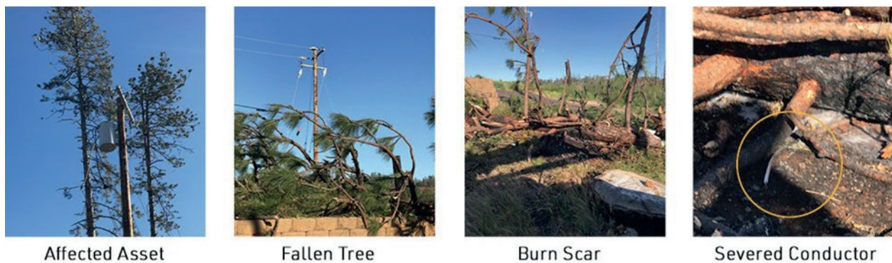
Figure 2: PG&E Covered Conductor Effectiveness – Example 1
