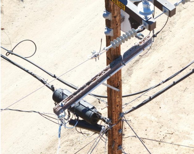
Figure JK- 2: P475444, 12/10/2021, Damaged Crossarm and view from below with no visible damage.
