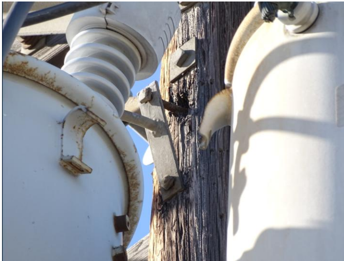
Figure JK- 3: P283191, 1/3/2022, Bolt coming out and view from below with no visible damage.
