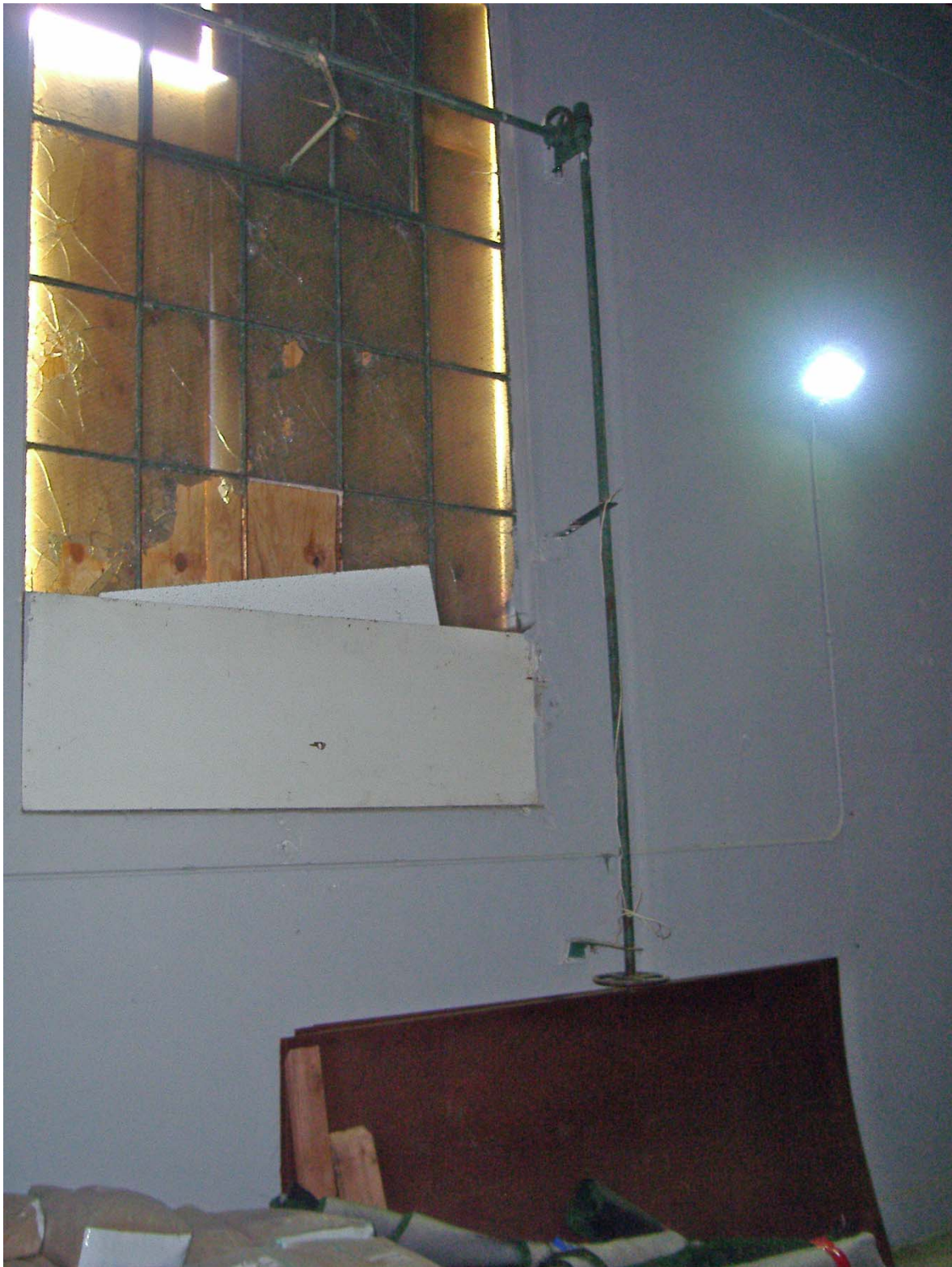
Example of Industrial Window with Crank-Handle Opener, East Elevation from Interior of Building (facing Southeast).
