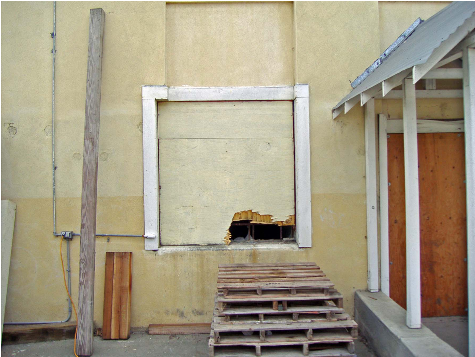
Altered Window on North Elevation of Ell (facing South).
