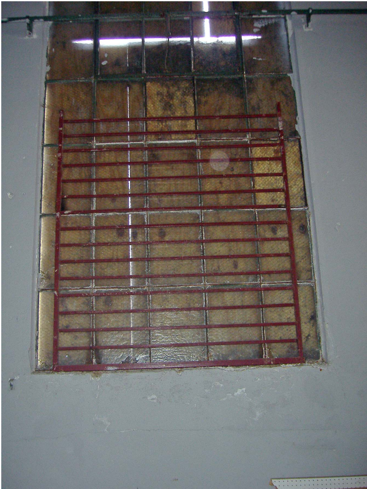
Detail of Industrial Window with Added Security Bars (West Elevation; facing West).
