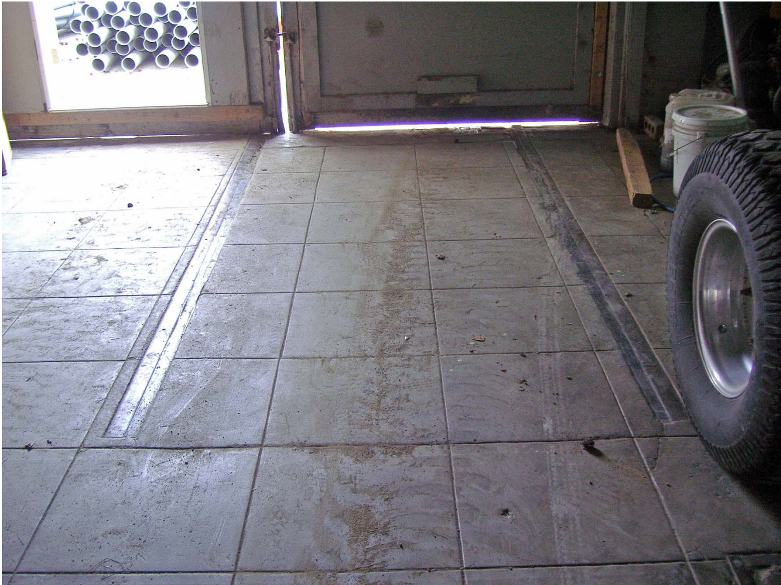
Detail fo Puoured Concrete Floor with Remnants of Rail Tracks (facing North).
