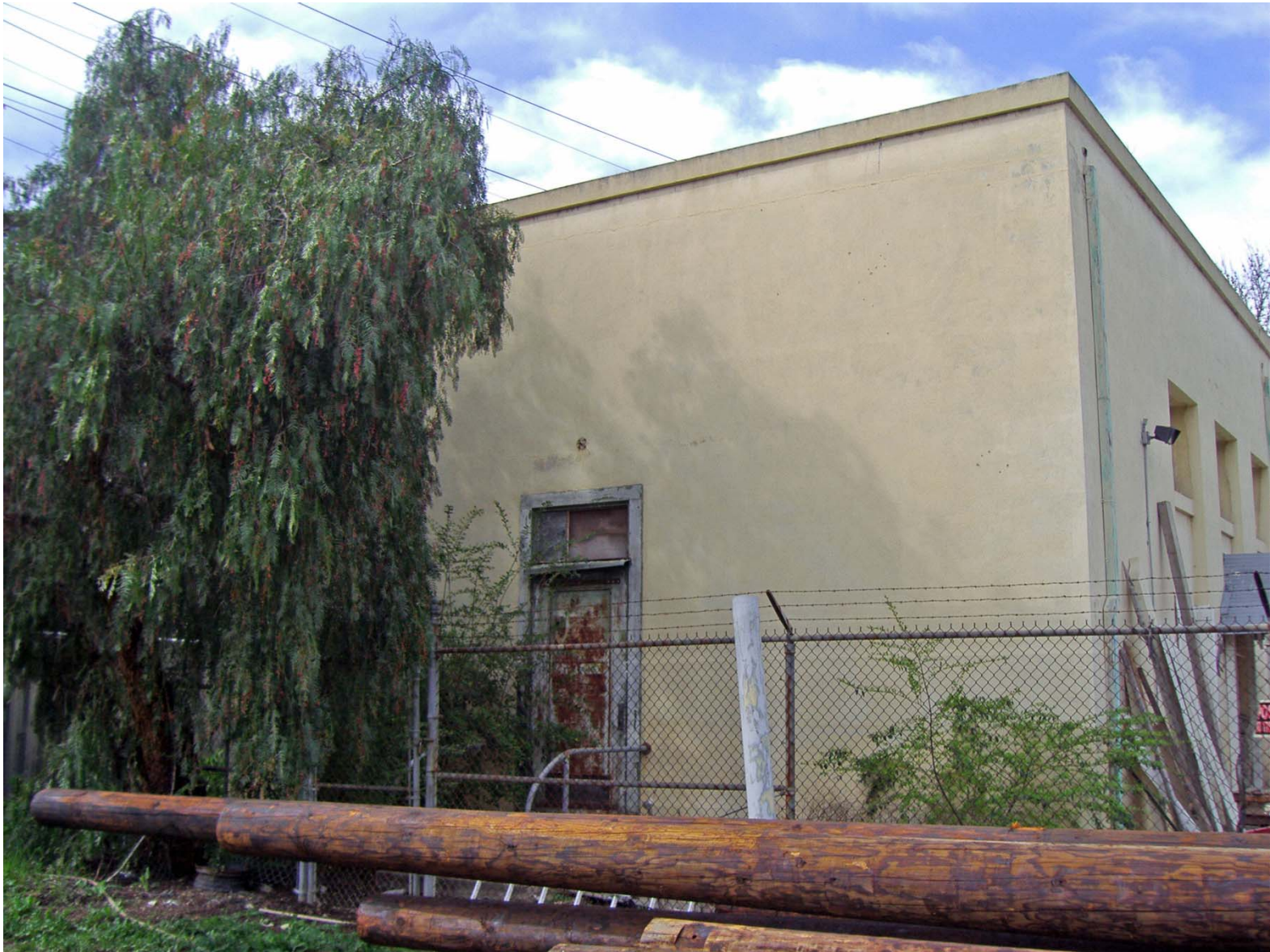
Overview of East Elevation (facing Southwest).
