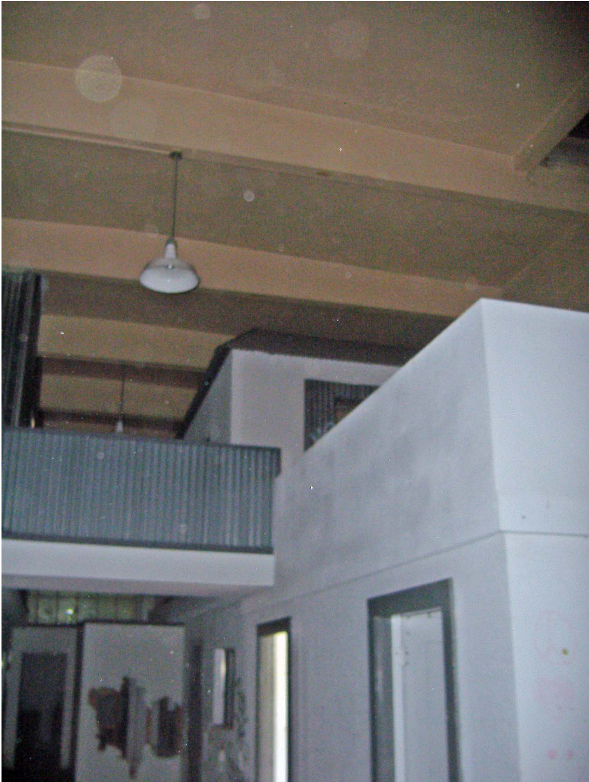
Overview of Second Story Offices (facing North/Northeast).
