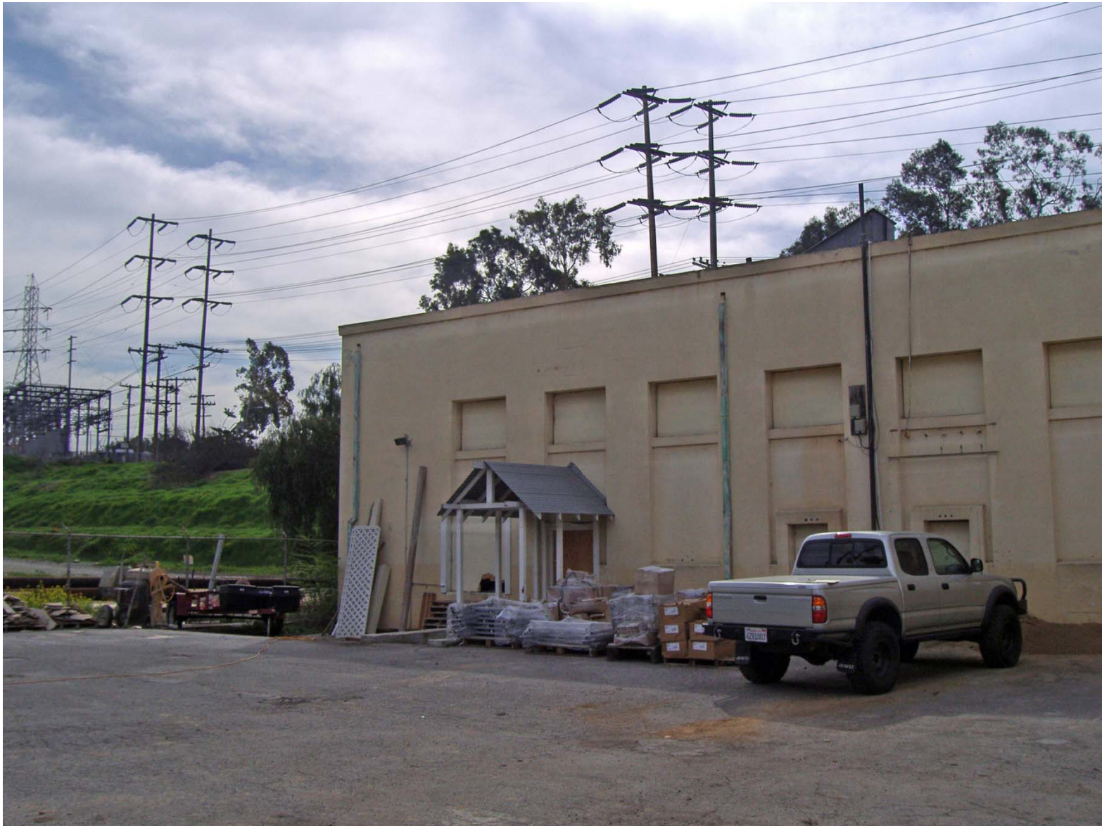
Overview of North Elevation of East Ell, SD G & E Building (facing Southeast).
