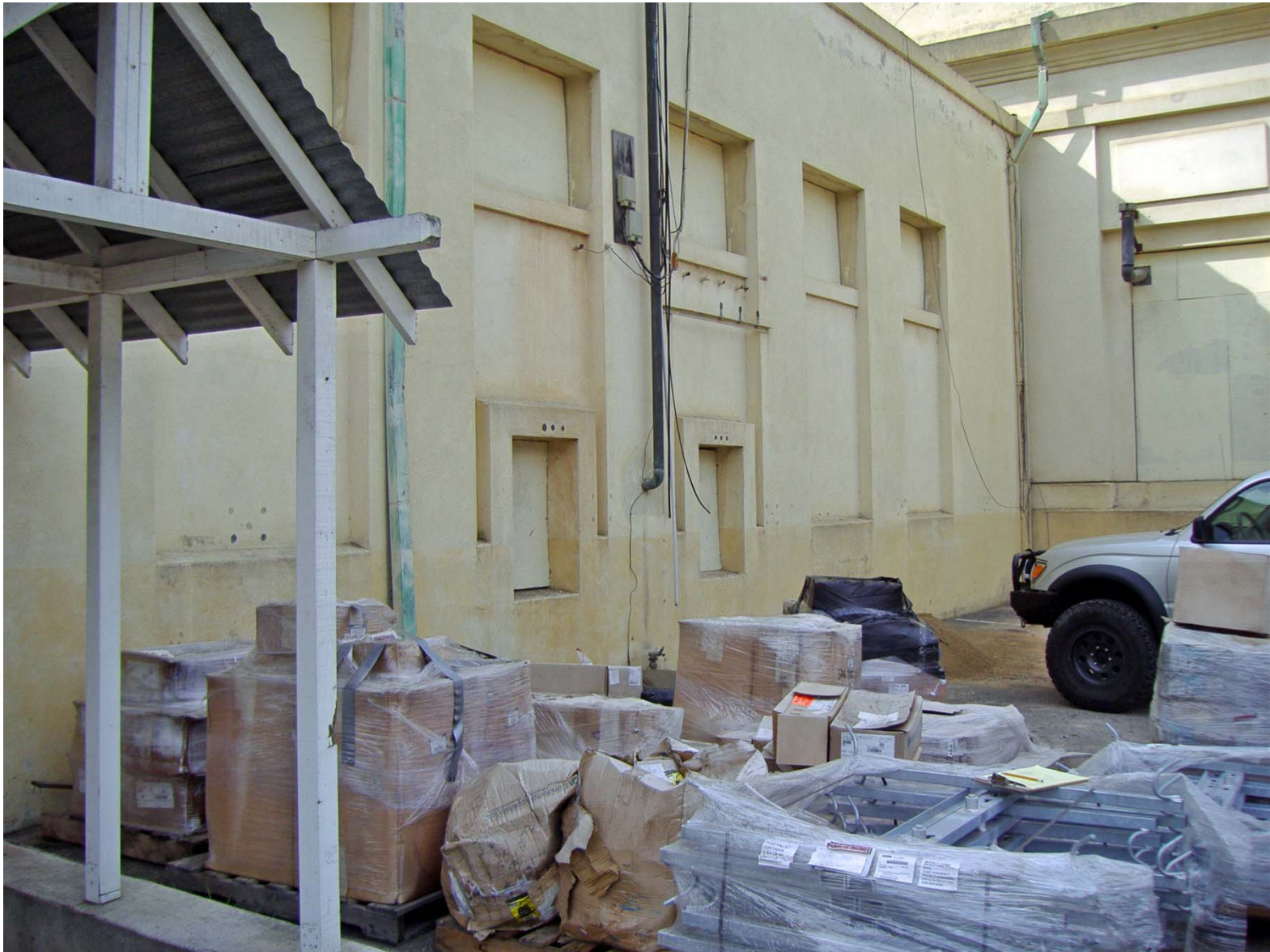
Overview of North elevation of Ell, SD G & E (facing West/Southwest).
