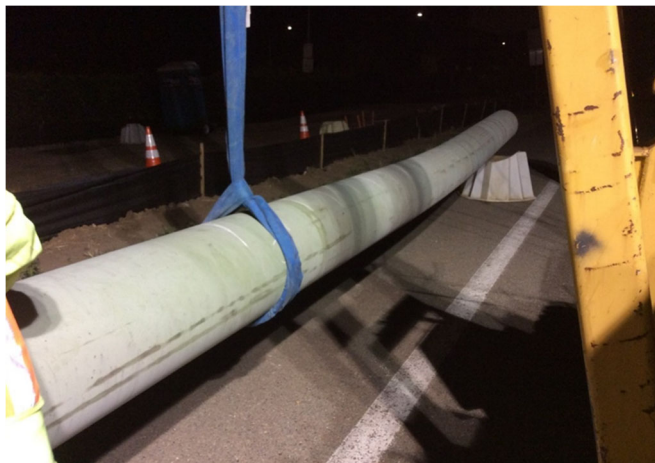
Figure 2: 16-inch Steel Pipe
