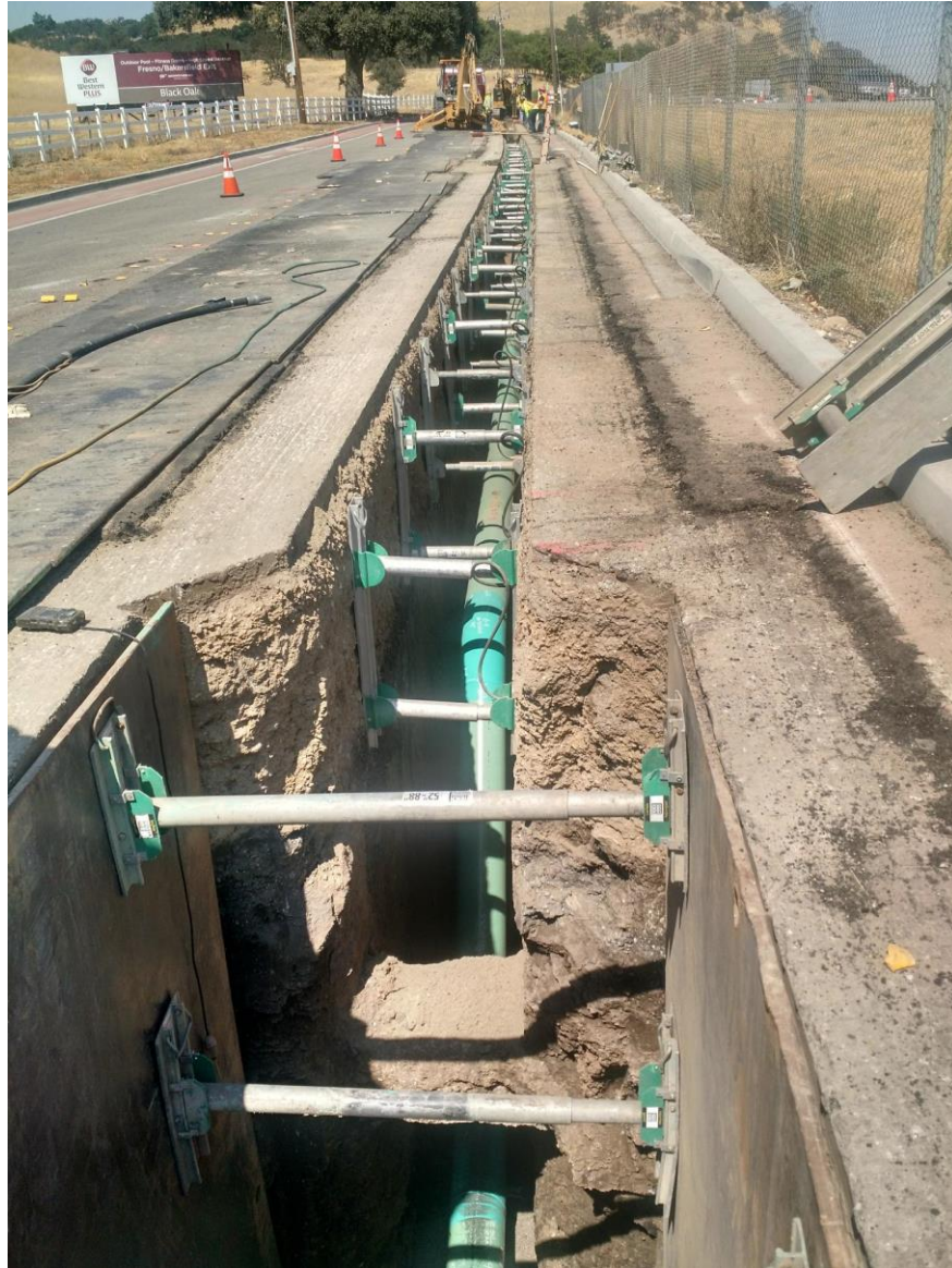
Figure 3: Trenching Along Vine Street
