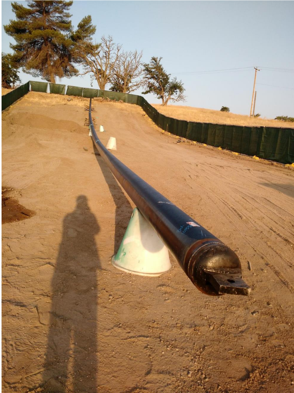
Figure 5: Preparation for the HDD Across Highway 101
