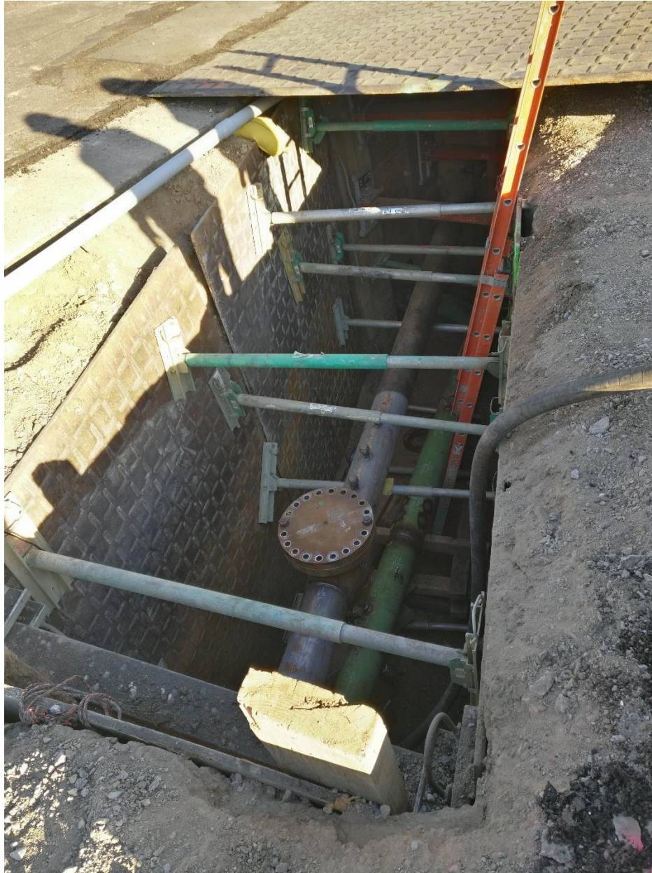
Figure 4: PCF Connecting the Old and New Pipeline
