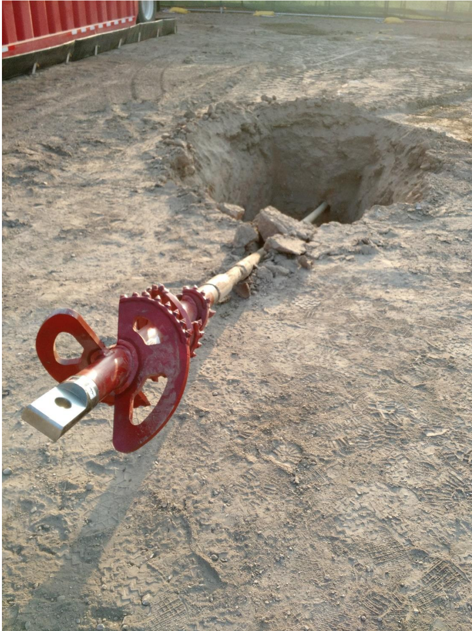
Figure 6: Back Reamer for HDD
