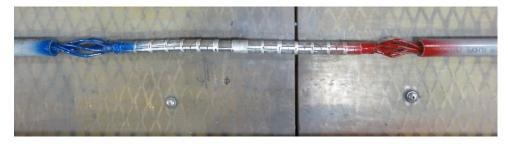
Figure 3-3: installed on 35 kV 1/0 AWG, 6/1 ACSR
