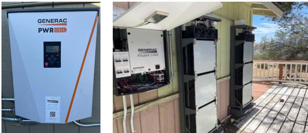
Figure 8-6: FPB Installation at Mobile Home Park Community
