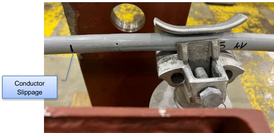
Figure 6-10: [REDACTED] - Typical 1/0 AWG ACSR (35 kV) Conductor Condition after Slip Test
