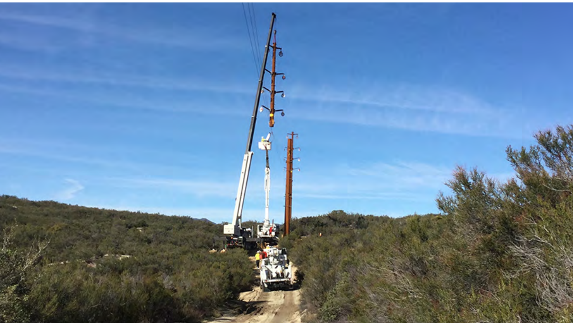
SDG&E crews replaced more than 2,300 wood poles with fire-resistant steel poles in the Cleveland National Forest.
