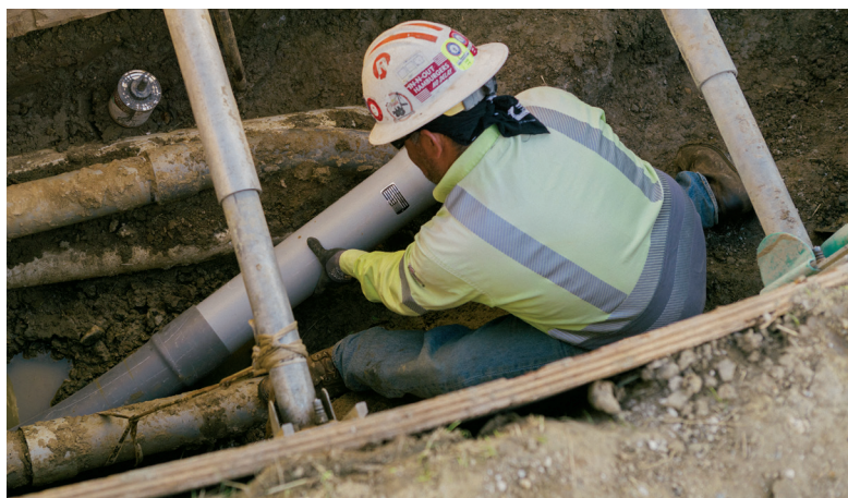
Undergrounding power lines.
