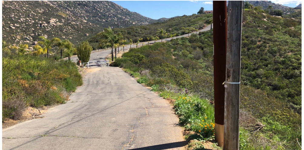
Older wood pole (right), being replaced by new steel pole (left).
