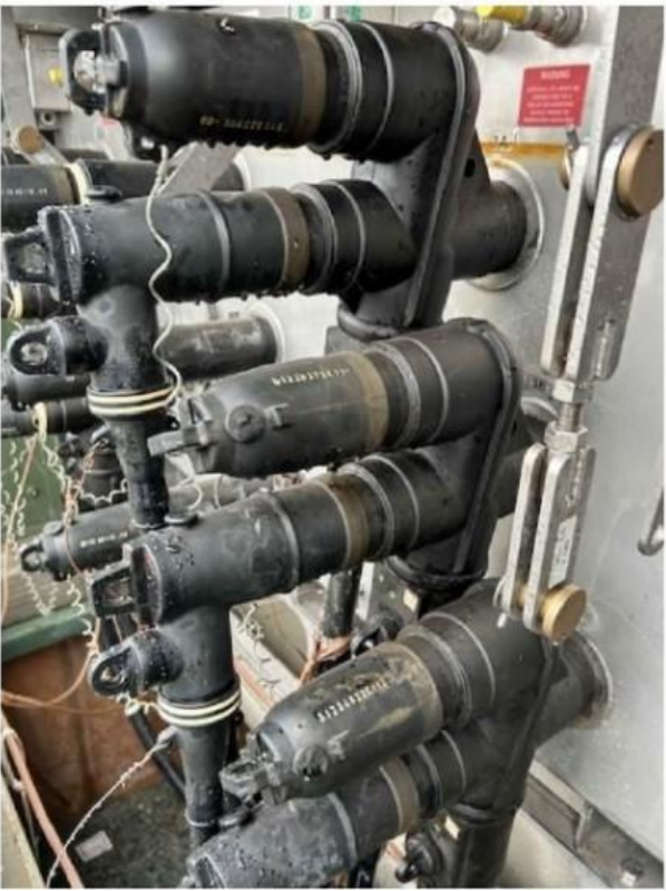
FIGURE 3 PHOTO 1-SIDE VIEW EQUIPMENT ELBOW 15KV R-800 DOUBLE INTERFACE
