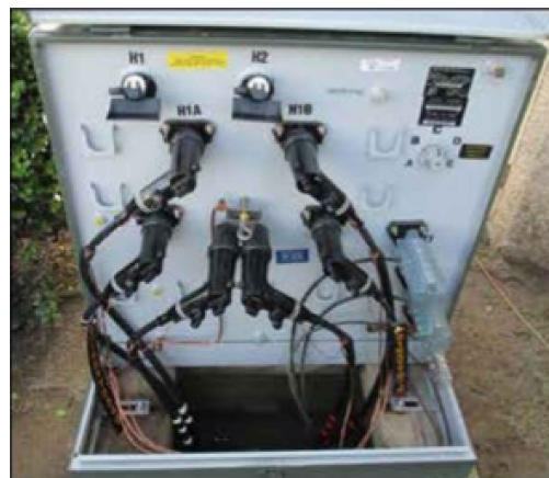
FIGURE 1 ACTUAL FIELD INSTALLATION
