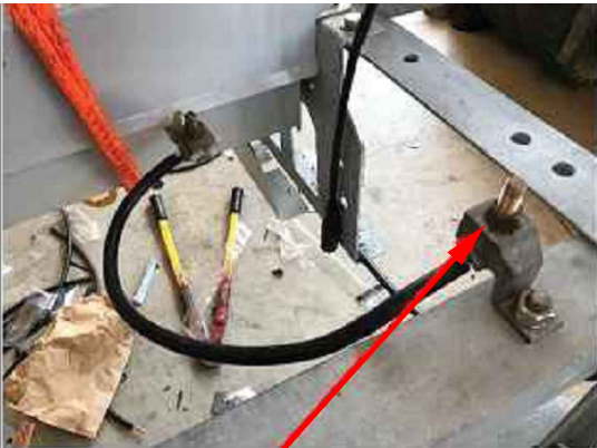
GROUND SWITCH FOR SWITCH FRAME
