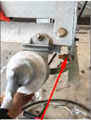
LOAD-SIDE ARRESTER GROUND
