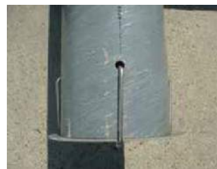
J-BOLTS ON OUTSIDE OF MODULE
