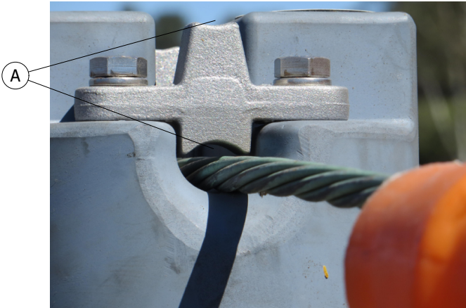
FIGURE 2 INCORRECT INSTALLATION
