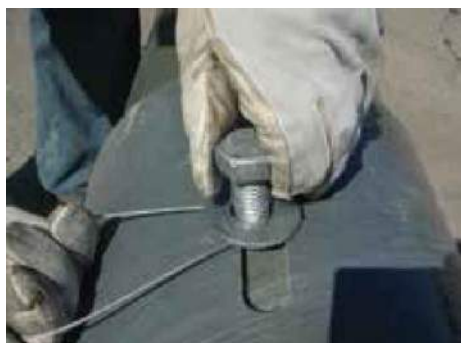
FIGURE 15 BOLT AND WASHER INSTALLATION
