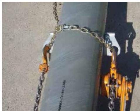
FIGURE 11 JACKING LUG SAFETY STRAP/CHAIN INSTALLATION
