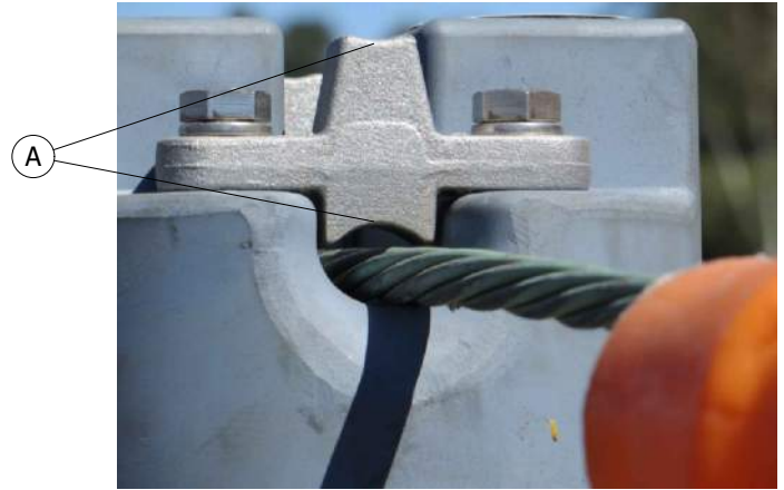
FIGURE 2 INCORRECT INSTALLATION
