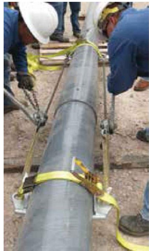
FIGURE 12 COME-ALONG INSTALLATION
