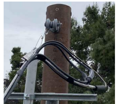
FIGURE 4 STORM SAFE FLEXIBLE BAIL ASSEMBLY
