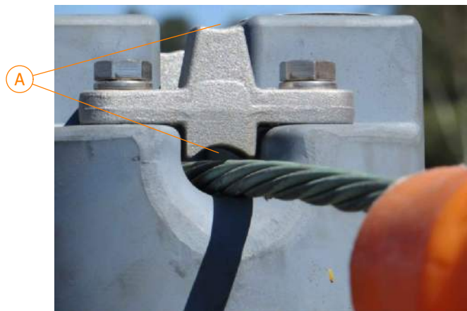
FIGURE 2 INCORRECT INSTALLATION
