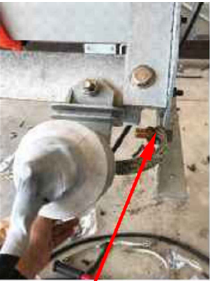
LOAD-SIDE ARRESTER GROUND
