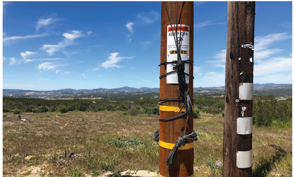
Older wood pole (right), being replaced by new steel pole (left).
