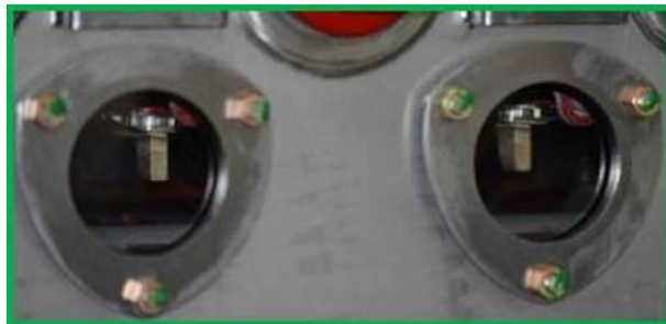
FIGURE 47 VISIBLE OPEN SHAFT (K2) "OPEN"
