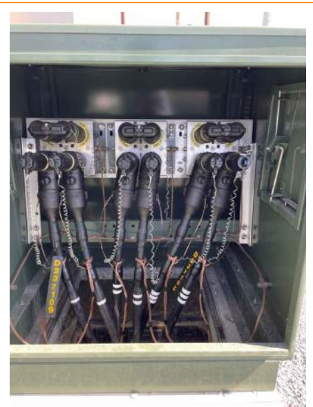
FIGURE 2 WITHOUT LOAD TRACKER FAULT INDICATORS
