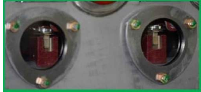
VISIBLE CLOSED SHAFT "CLOSED"
