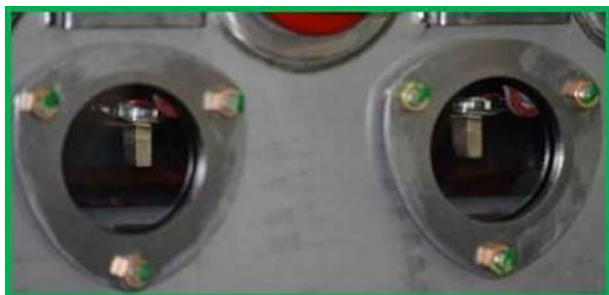
FIGURE 47 VISIBLE OPEN SHAFT (K2) "OPEN"
