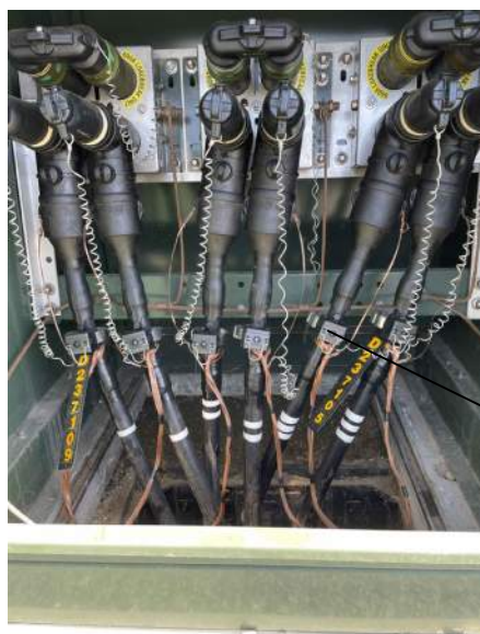
FIGURE 2 WITH LOAD TRACKER FAULT INDICATORS
