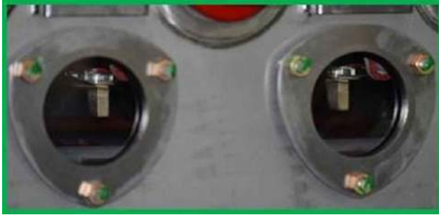
VISIBLE OPEN SHAFT "OPEN"
