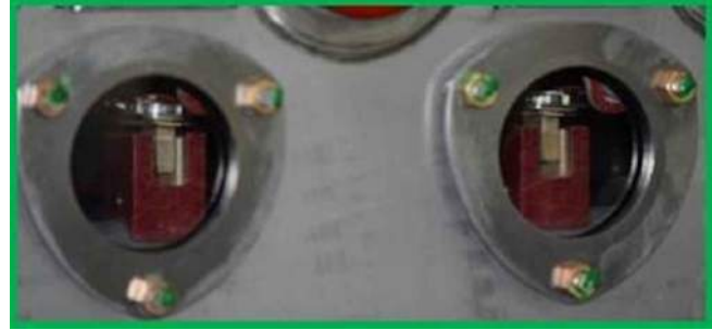
VISIBLE CLOSED SHAFT "CLOSED"
