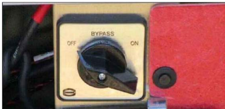
FIGURE 5 BYPASS SWITCH (E)
