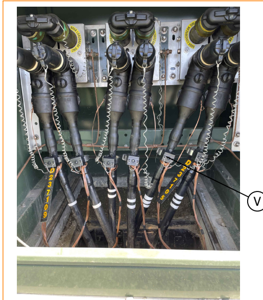
FIGURE 2 WITH LOAD TRACKER FAULT INDICATORS
