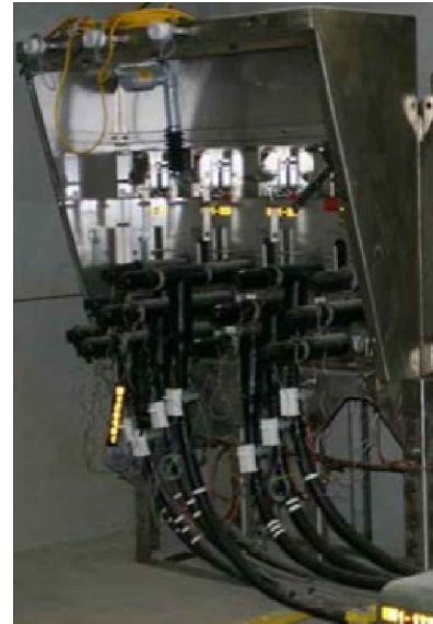
FIGURE 6 4-WAY MANUAL WITH (III) LINEAR ACTUATOR
