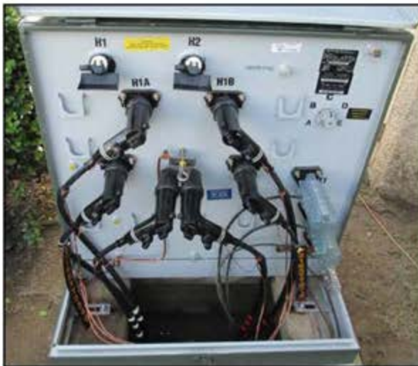
ACTUAL FIELD INSTALLATION OF SKETCH IN THE DEPICTION ON THE TOP.
