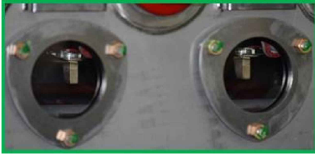
VISIBLE OPEN SHAFT "OPEN"
