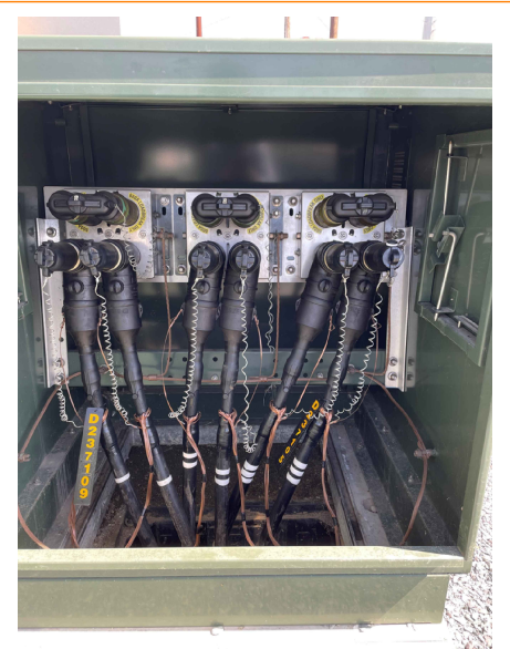
FIGURE 2 WITHOUT LOAD TRACKER FAULT INDICATORS
