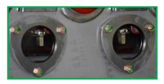
FIGURE 47 VISIBLE OPEN SHAFT (K2) "OPEN"
