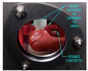
VISIBLE OPEN SHAFT "OPEN", ISOLATED AND VISIBLE
