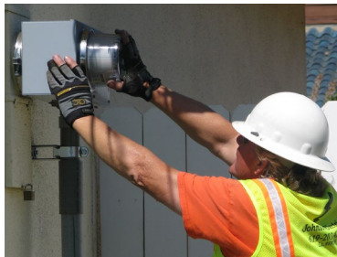
Crews will need to access meter service panels so they are ready for new underground service.
