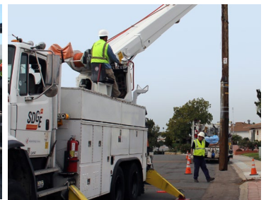
Partial, temporary street closures will be needed when crews remove poles.
