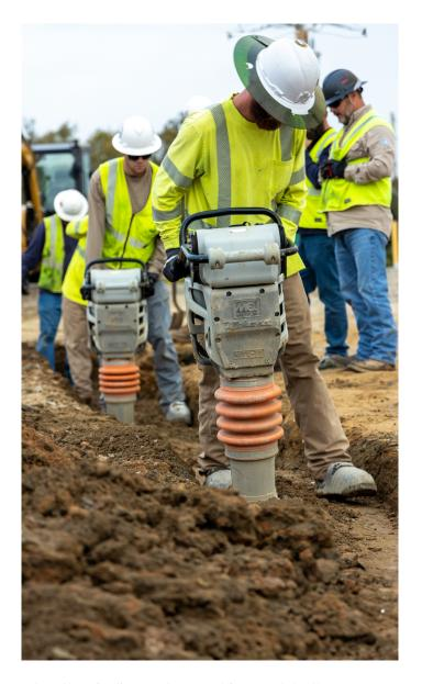
When the pipeline replacement is complete, the excavated sites are "back-filled" by returning the removed soil into the trench, and later graded and restored as closely as possible to their preconstruction condition. Any needed street or property repairs are also made.
