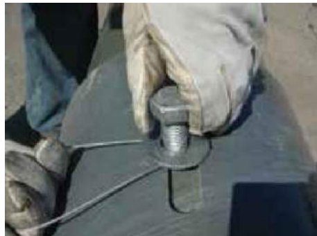
FIGURE 15 BOLT AND WASHER INSTALLATION
