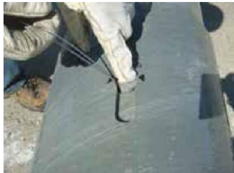
FIGURE 14 BLIND NUT INSTALLATION
