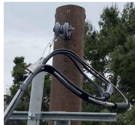
FIGURE 4 STORM SAFE FLEXIBLE BAIL ASSEMBLY
