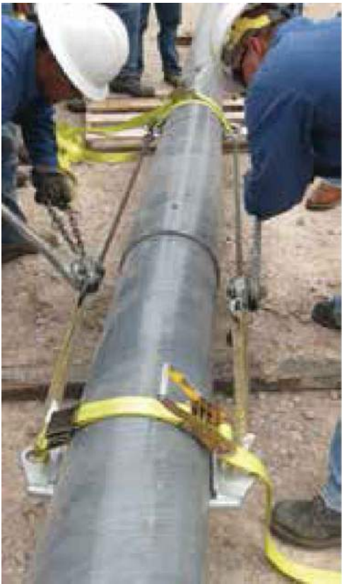
FIGURE 12 COME-ALONG INSTALLATION
