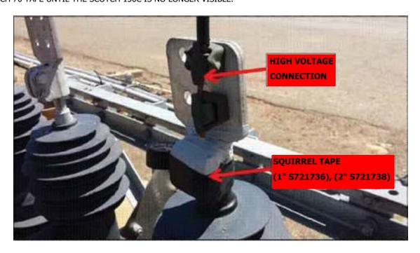
4. REATTACH THE EXTERNAL VOLTAGE SENSORS BACK TO THE VERTICAL NEMA-4 BUSHINGS USING A RATCHET WRENCH AT A TORQUE SETTING OF 25 FT-LBS. MAKE SURE TO RECONNECT THE SMALL CANNON PLUG FROM THE BOTTOM OF EXTERNAL SENSORS INTO THE RECEPTACLES FOUND ON THE FRAME OF RECLOSER FOR EACH PHASE.
