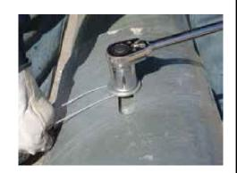
FIGURE 15 **BOLT AND WASHER INSTALLATION**
