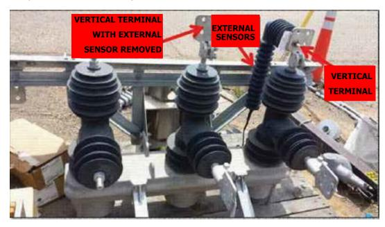
2. ONCE THE EXTERNAL SENSORS ARE REMOVED, APPLY THE SCOTCH 70 SELF FUSING TAPE (S720384) TO THE BASE OF EACH NEMA-4 VERTICAL TERMINAL WITH ENOUGH WRAPS TO COVER THE ENTIRE METAL SURFACE. SELF-FUSING TAPE COMES IN TWO SIZES: 1 INCH (S721736) AND 2 INCH (S721738).
