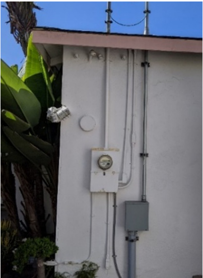
FIGURE 4: Loop & Bond Underground Service Connection - Rear Lot Panel
