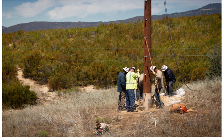
Crew replacing a wood pole with a fire-resistant steel pole.
