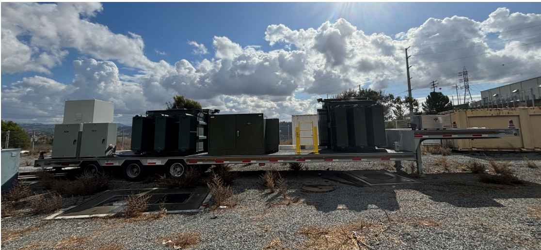
Figure 2. Photo Demonstrating Companion Trailer Configuration
