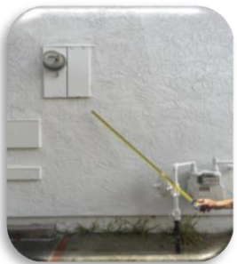
If electric meter panel is near gas meter, tape measurement proving gas is out of electric meter clearance requirement
