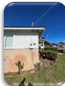
Panel location showing at least 5' of space to the left and right of meter location, from ground level to the roof & point of attachment, and working space in front of meter location
