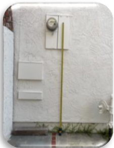
Measurement showing meter panel height from ground to center line of meter
