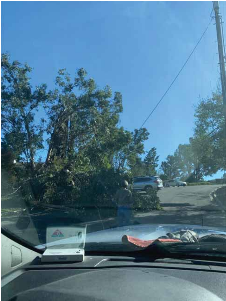
Figure 24 - Item #2 P108167 Broken Pole
